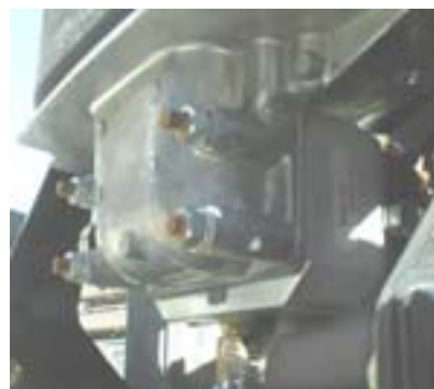
Figure 41. Venturi mixer body installed between the air-cleaner inlet and an existing carburetor
