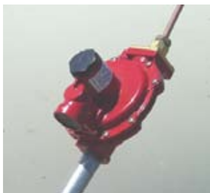
Figure 20. First- or primary-stage pressure regulator used in vapor service
