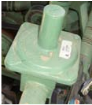
Figure 22. Pilot pressure regulator used in vapor withdrawal systems
