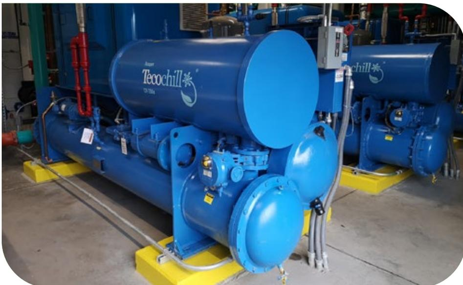
A marijuana grower in Douglas, Massachusetts, installed three Tecochill propane-driven chillers to meet the facility's large cooling and dehumidification needs without the need for electric utility upgrades.
