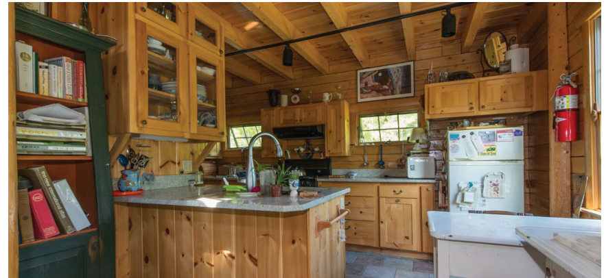
Ward Cedar Log Homes of Houlton, Maine, supplied the northern white cedar for siding and purlins and pine for interior walls. The galley kitchen, designed for greater efficiency, includes a three-burner stove, broiler, and oven fueled by propane.
