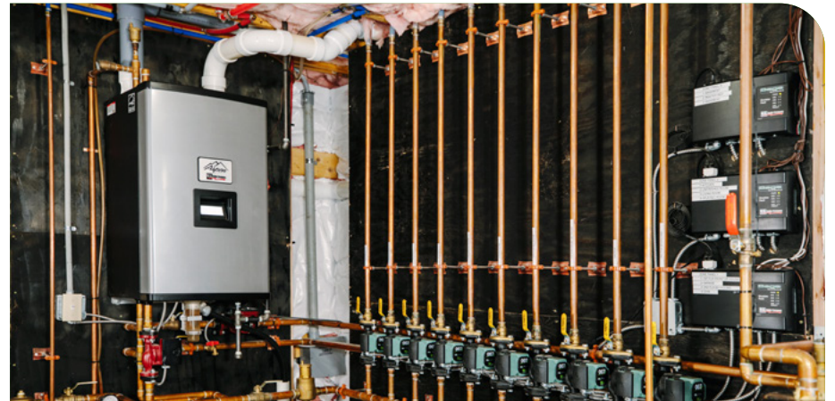
Long's heating system includes a condensing boiler, 10 hydronic zones, and two heat pumps for use in the shoulder seasons. A 70-gallon indirect water tank provides plenty of hot water for the multi-head shower in the primary bedroom suite.
