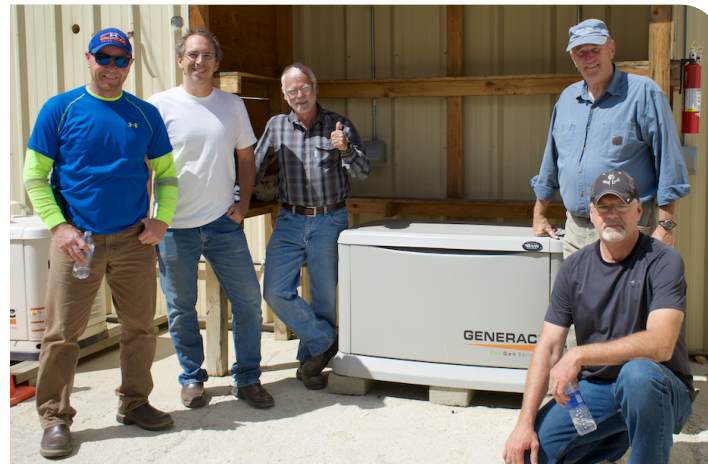
Midas Gold staff pose with the EcoGen propane generator. From left to right: Chuck Eilers, Lead Equipment Operator; Kelley Dagley, Dagley LLC; Bob Barnes, COO; Richard Moses, Field Operations Manager; Layne Mouritsen, Field Operations Supervisor.
